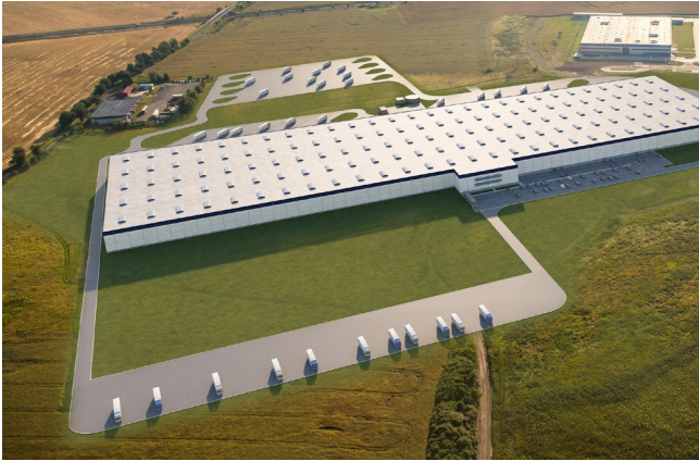
Distribution centre Tchibo, Cheb, Czech Republic LOGICROOF V-RP 1.5 mm | 65.000 m 2
