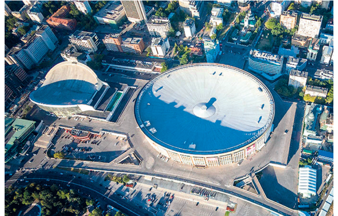
Olympic Stadium, Moscow, Russia LOGICROOF V-RP FB 1.8 mm | 40.000 m 2
